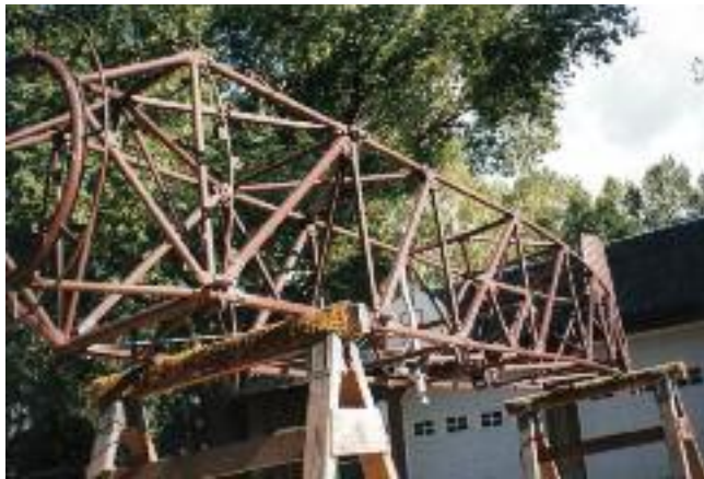
When all eight basic structures including their welded steel engine mounts were complete and primed, they were placed in the painting fixture right, to receive their final aluminum coating.
